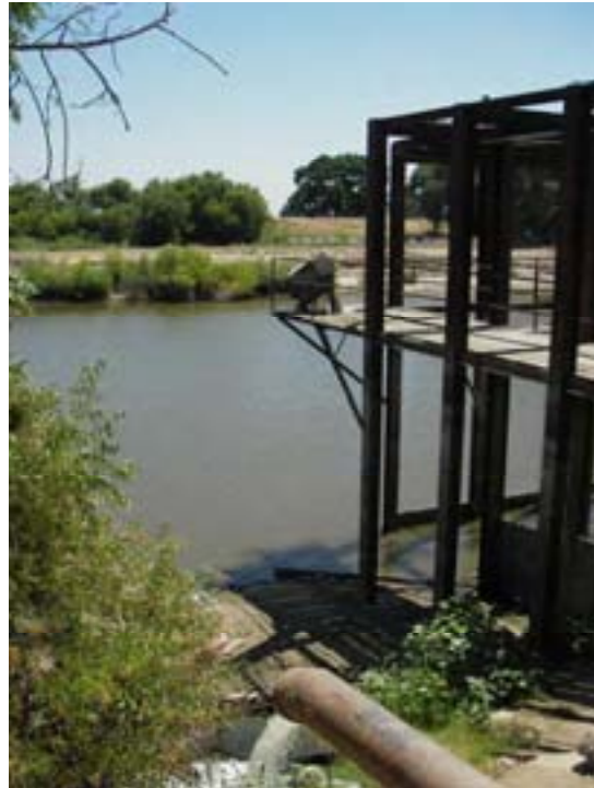
Figure 5: Patterson irrigation district intake structure on San Joaquin river, DO-07.
