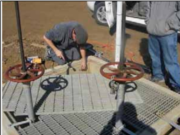
DO-130 Marshall Rd Res Entrance Jeremy Hanlon mounting the sonde to the side of the concrete structure.
