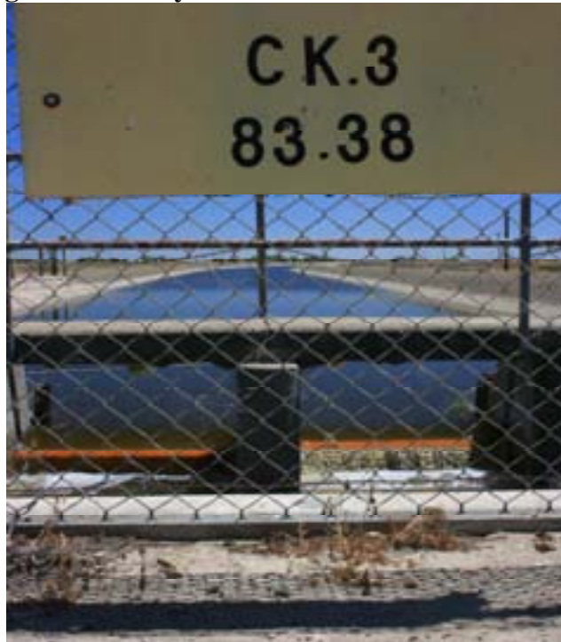
Figure 20: Check Station 3 water was flowing over boards, sonde profile was done from concrete bridge immediately in front of boards.
