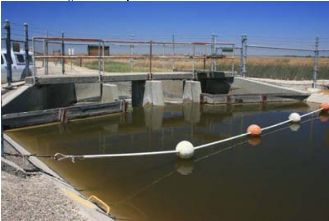
Figure 21: Check Station 3 water was flowing over boards, sonde profile was done from concrete bridge immediately in front of boards.
