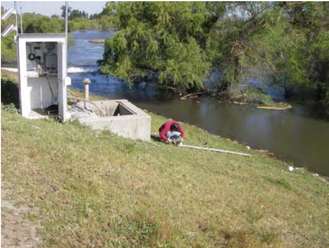
Figure 9: Kyle Kearney inspecting the damage to Ramona Lake Drain flow station. San Joaquin River flooding backed up into the culvert and decommissioned the station.
