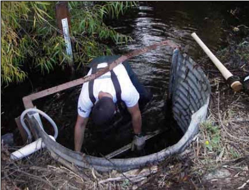
DO-60 Moffit 1 South Jesse Merkel cleaning off the weir boards.
