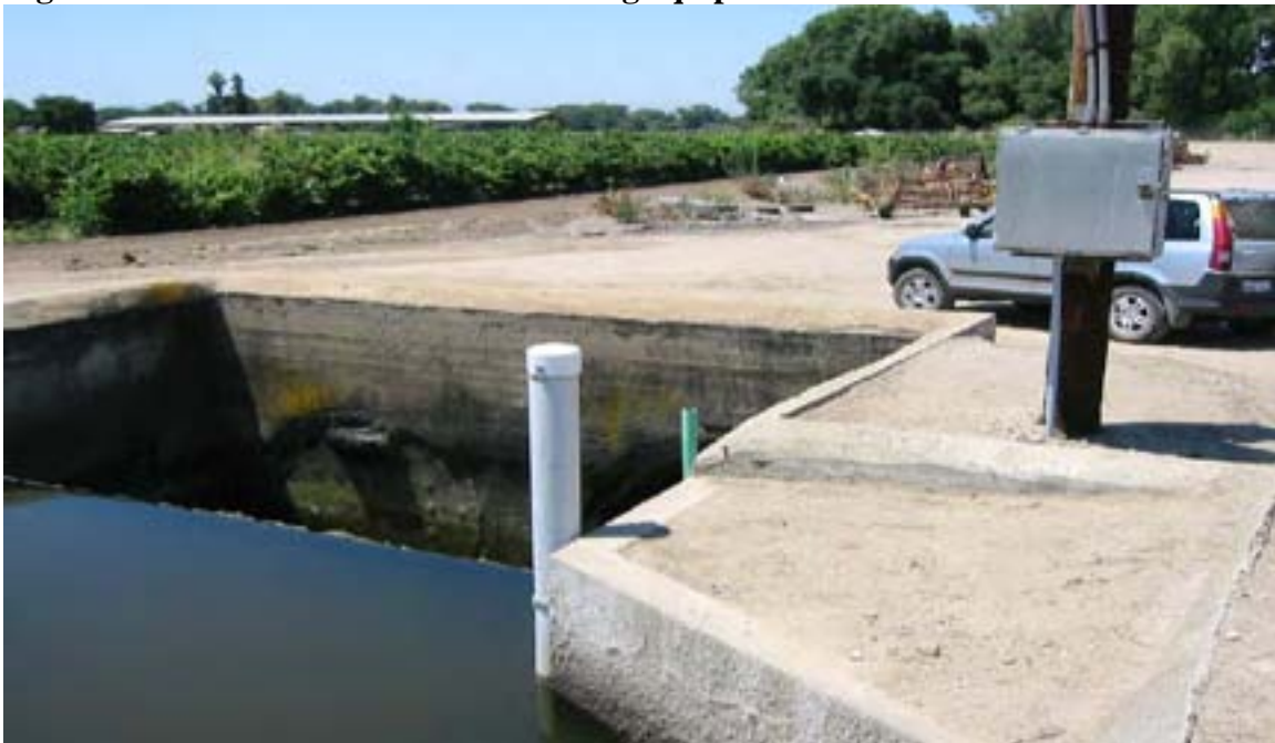
Figure 20: Weir structure and monitoring equipment at MID Lateral 6.
