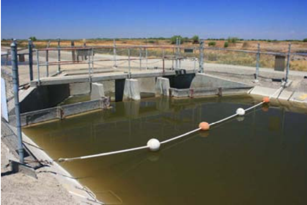
Figure 24: Check Station 4 water flowing over boards, strong current made it difficult to keep instrument in place.
