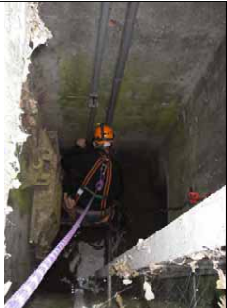
DO-64 Moran Drain Chris Linneman (Summers Engineering) drilling anchors into the concrete to stabilize bubbler pipe.
