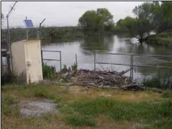
DO-61 Deadmans Slough Photo of debris placed over the weir structure by beavers.
