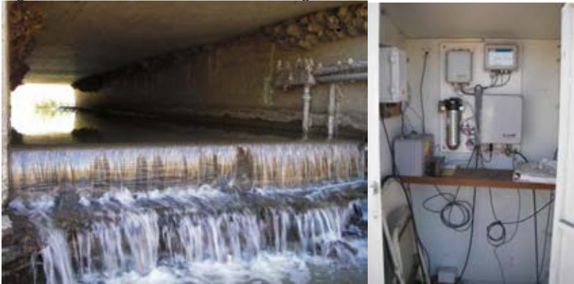
Figure 15: Weir and flow station shed at Ingram Creek.
