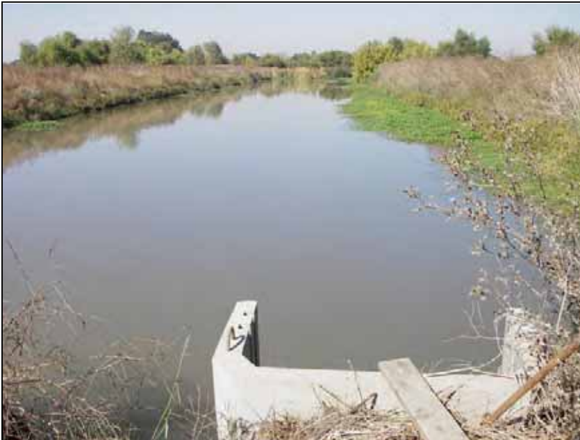
DO-35 Westley Wasteway Weir structure confining the water in a pond at Westley Wasteway.
