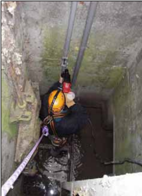
DO-64 Moran Drain Chris Linneman (Summers Engineering) drilling anchors into the concrete to stabilize bubbler pipe.
