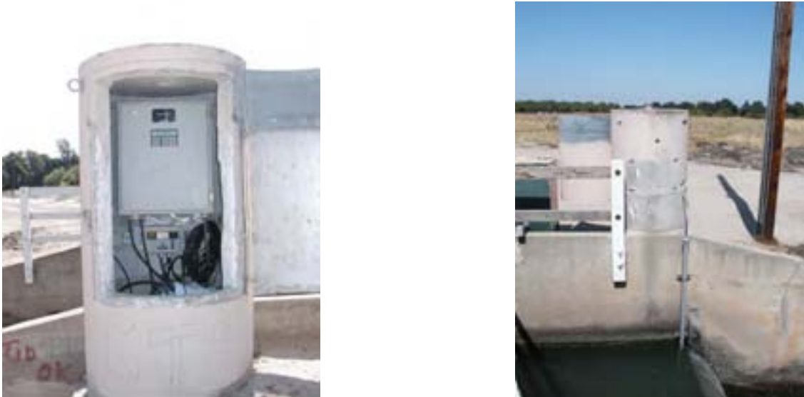
Figure 23: (left) Sierra Controls SCADAPACK and (right) weir structure at TID Highline Canal.
