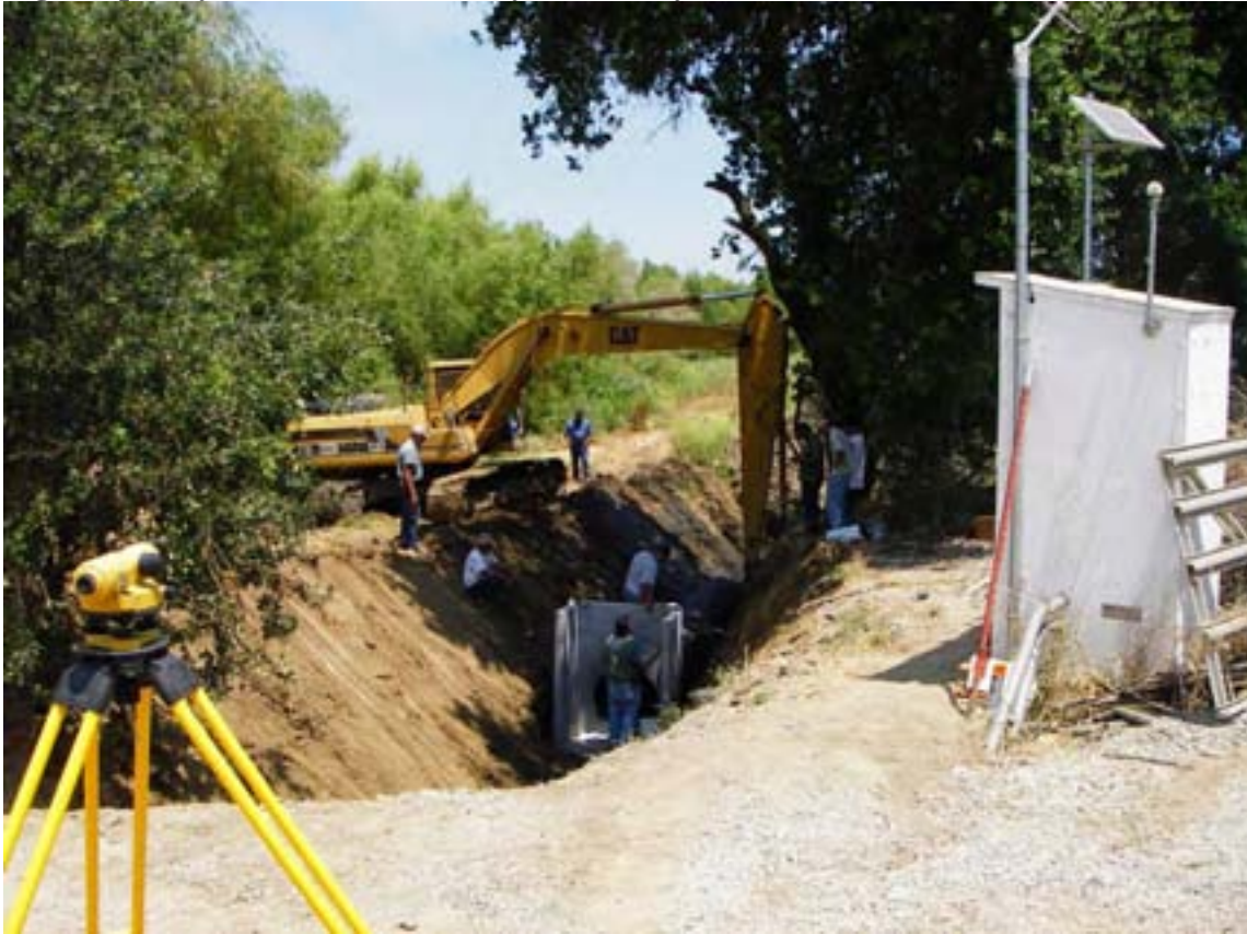
Figure 12: Irrigation district installing a new weir structure and culvert to provide higher quality flow data at Westley Wasteway.
