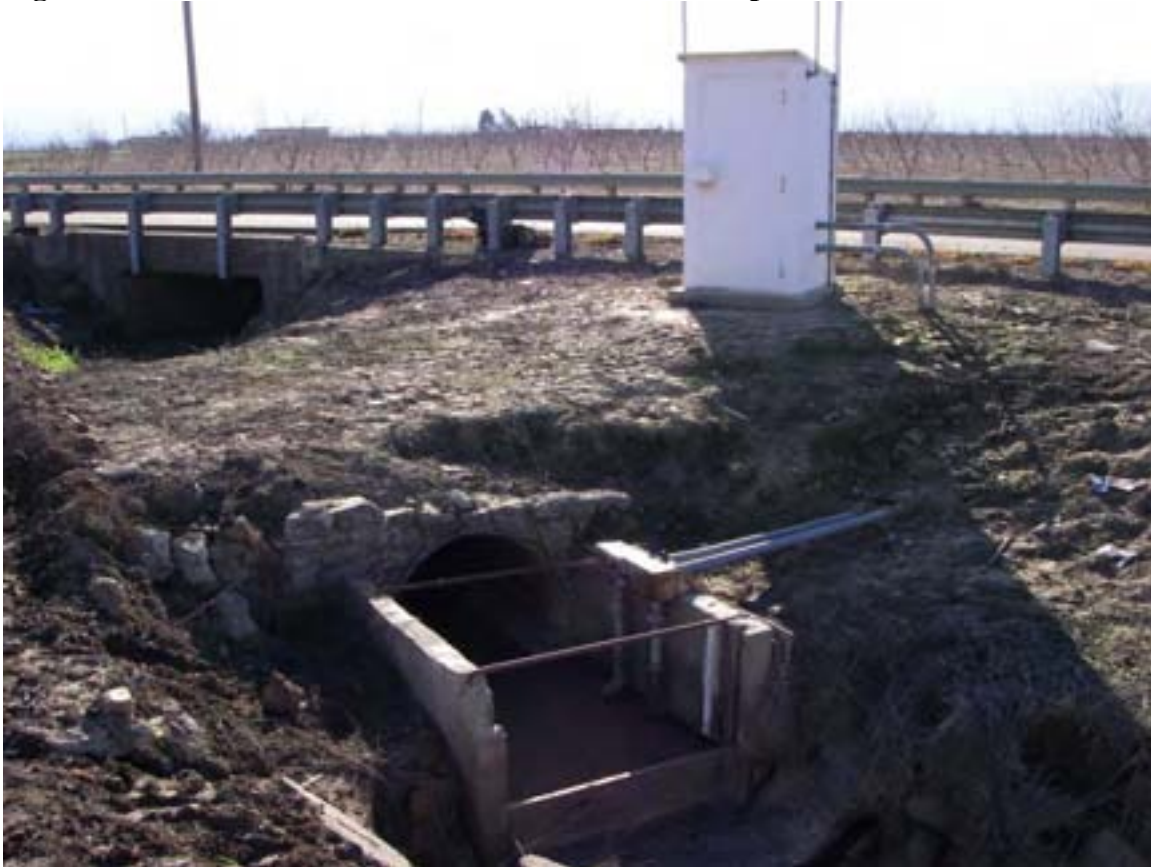
Figure 14: Flow station shed and weir structure at Hospital Creek.
