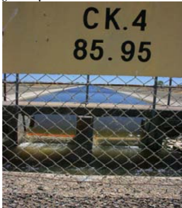
Figure 23: Check Station 4 water flowing over boards, sonde profile was performed from concrete bridge directly in front of weirboards.
