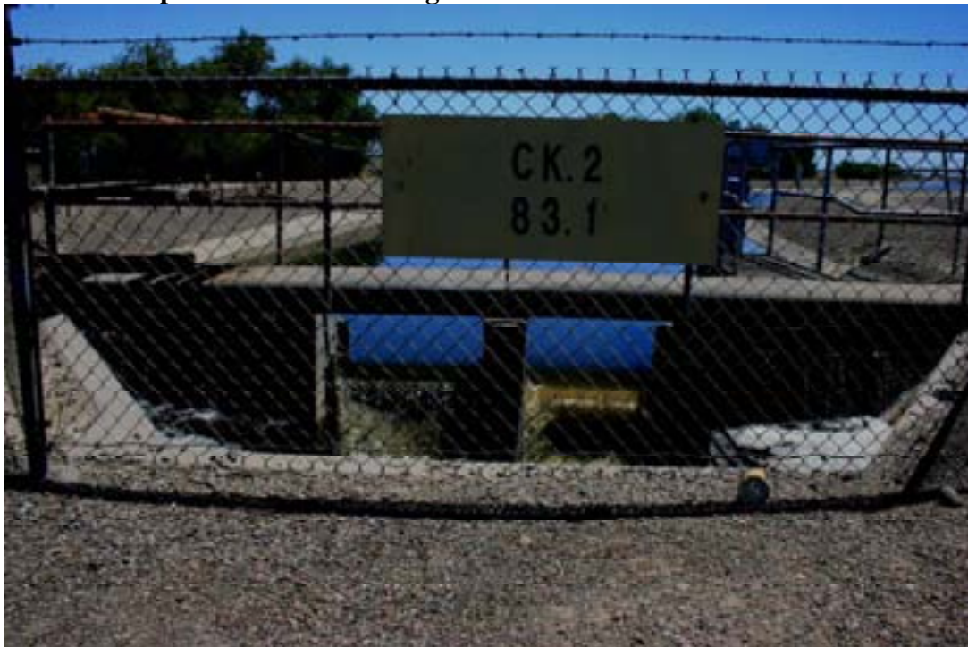
Figure 17: Check Station 2 water had begun to flow over the boards, sonde profile was done from platform where stilling well is located.
