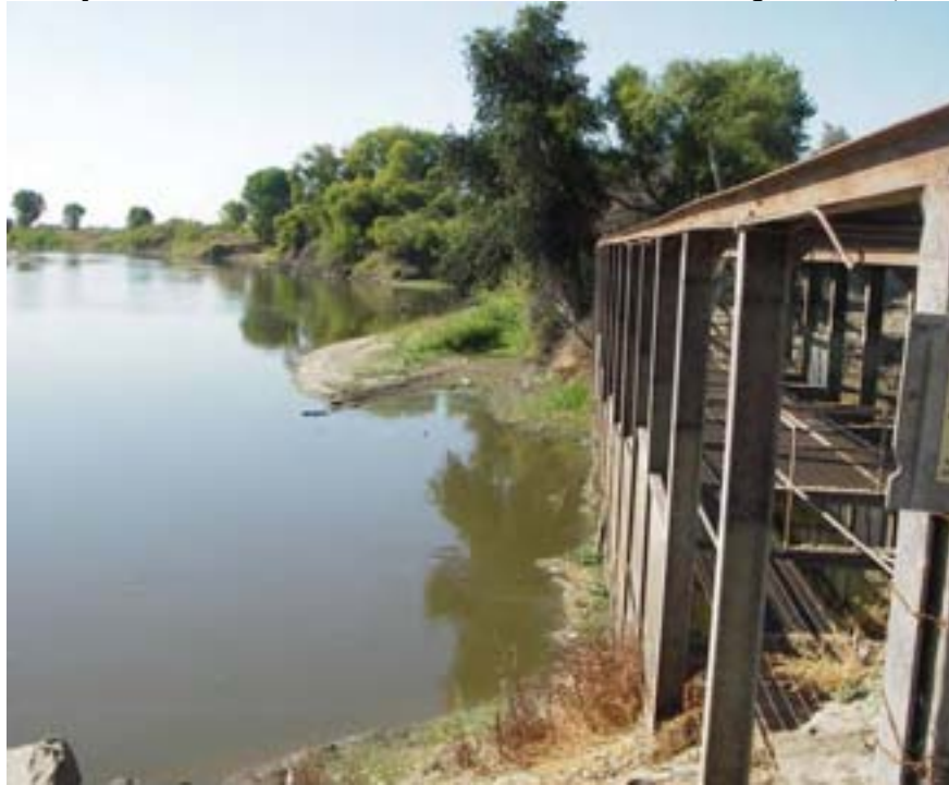
Figure 4: Elsolyo water district intake structure on San Joaquin river, DO-06.
