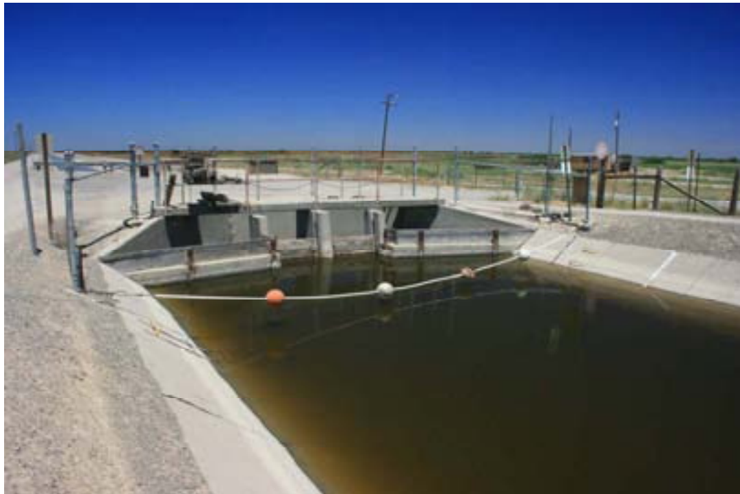
Figure 15: Check Station 1 had leaky boards, sonde profile was performed from wall near boards.
