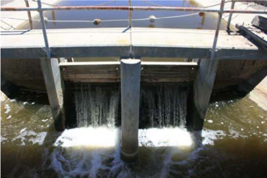
Figure 14: Check Station 1 had leaky boards, sonde profile was performed from wall near boards.
