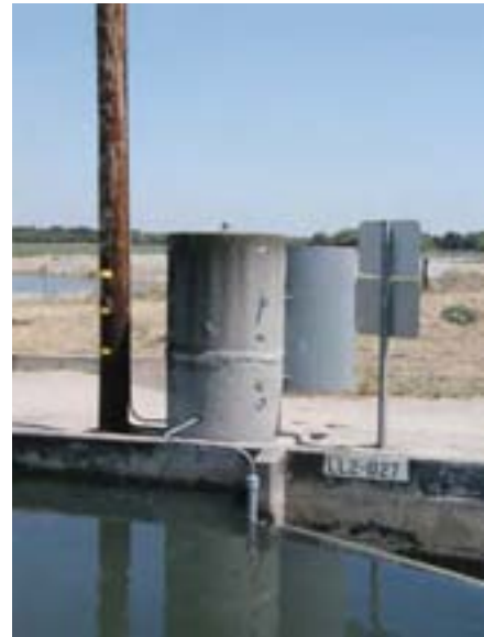
Figure 24: (left) Flow monitoring equipment and (right) weir structure at TID Lateral 2.
