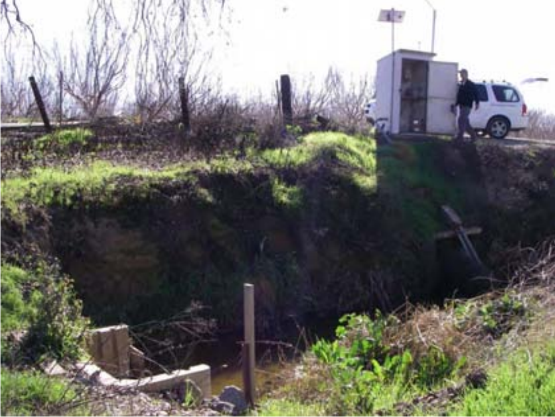
Figure 13: Current setup at Westley Wasteway. Weir structure and pond with bubbler system provide high quality flow data with very few problems.
