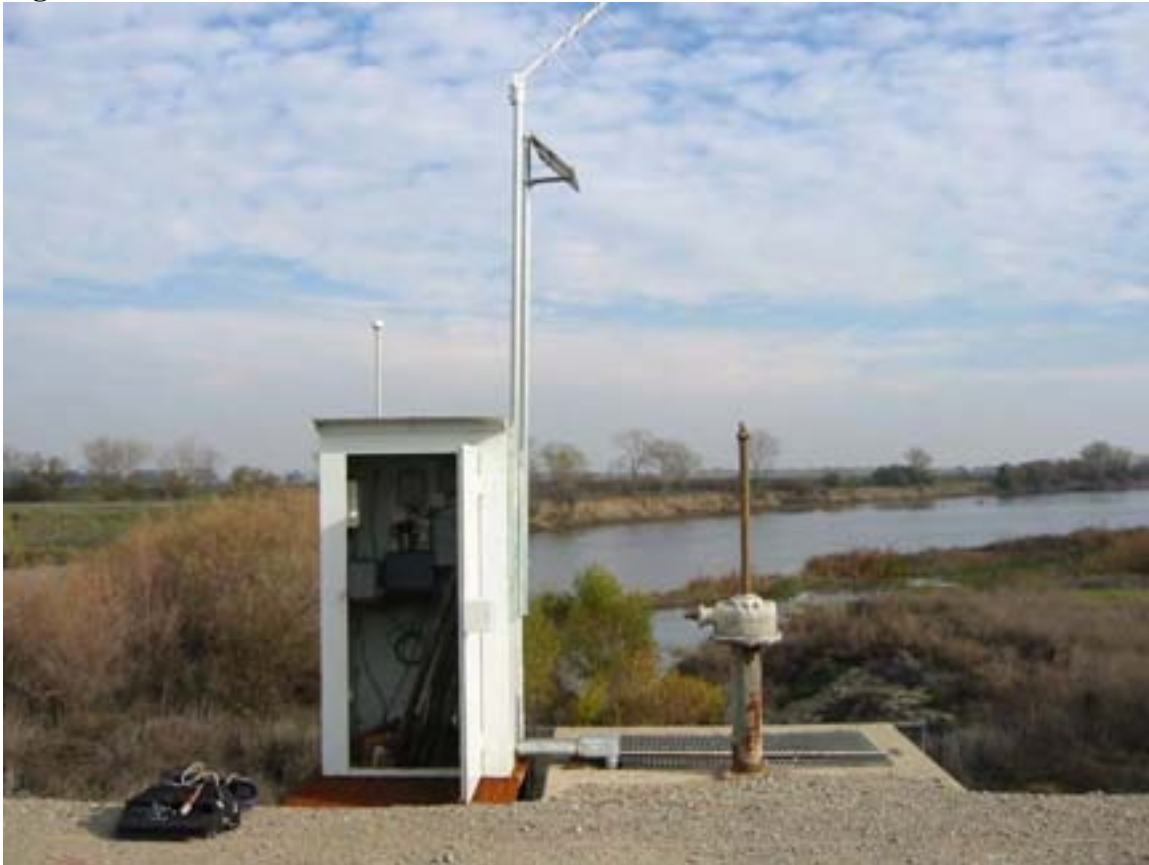
Figure 17: Flow station shed and manhole at New Jerusalem Drain.
