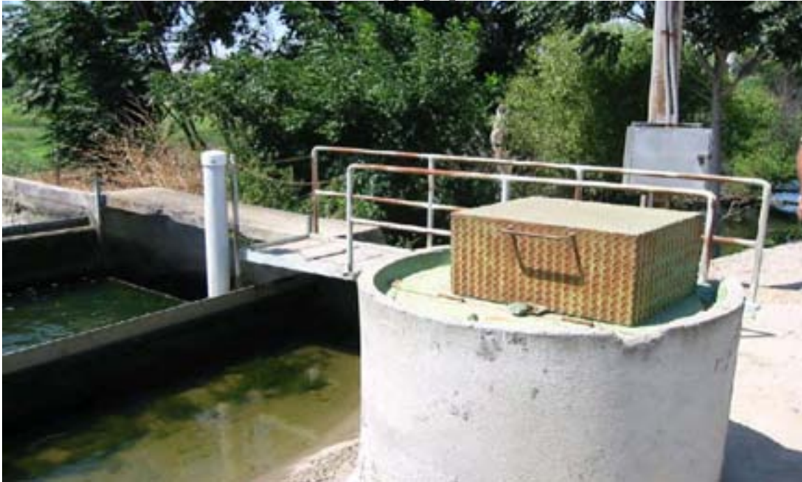
Figure 19: Weir structure and monitoring equipment at MID Lateral 5.
