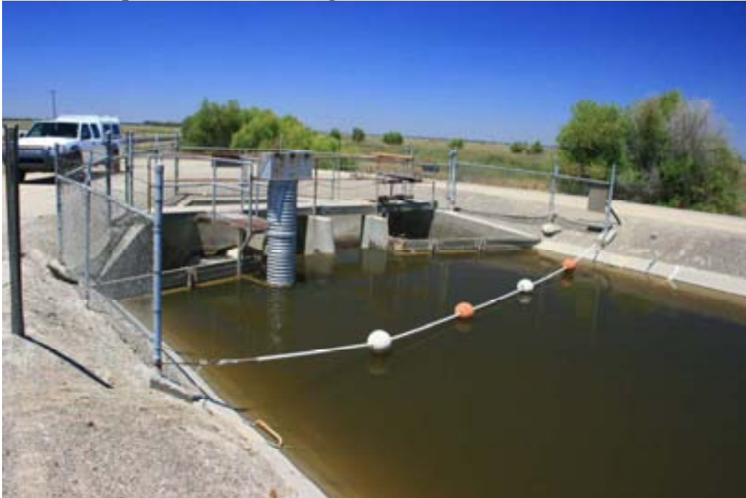
Figure 18: Check Station 2 water had begun to flow over the boards, sonde profile was done from platform where stilling well is located.
