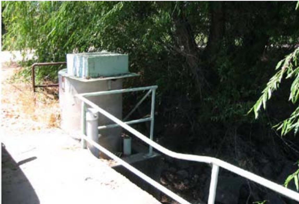
Figure 21: Stevens chart recorder and YSI EC probe next to bridge over the weir structure at MID Miller Lake Outfall.
